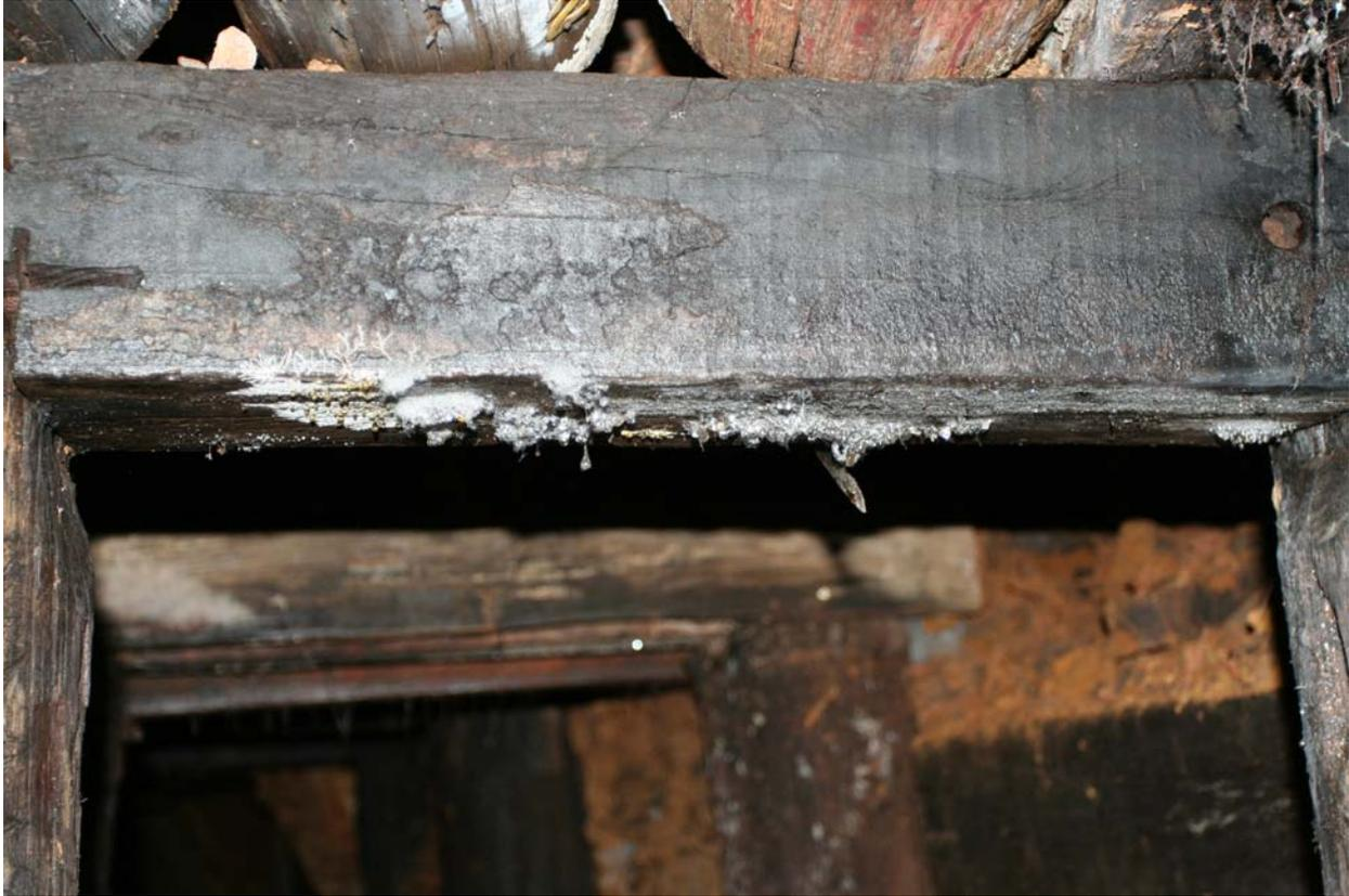
**View of the Marshall Mine Shoring. Note the Peg Type Connection Between the Cross Tie and Vertical Support. Ceiling Shoring Is Made from De-barked Logs. Photo by W.B. Carah**
